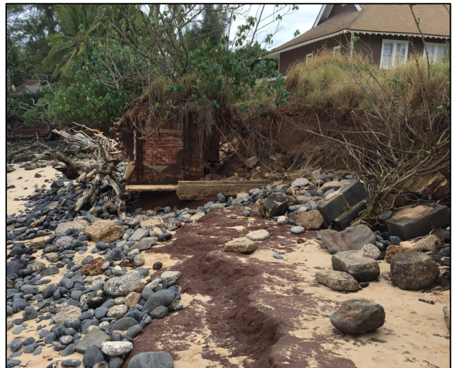
Figure 2: Photograph taken in January 2019, showing the eroded shoreline with exposed debris and fallen headstones.
